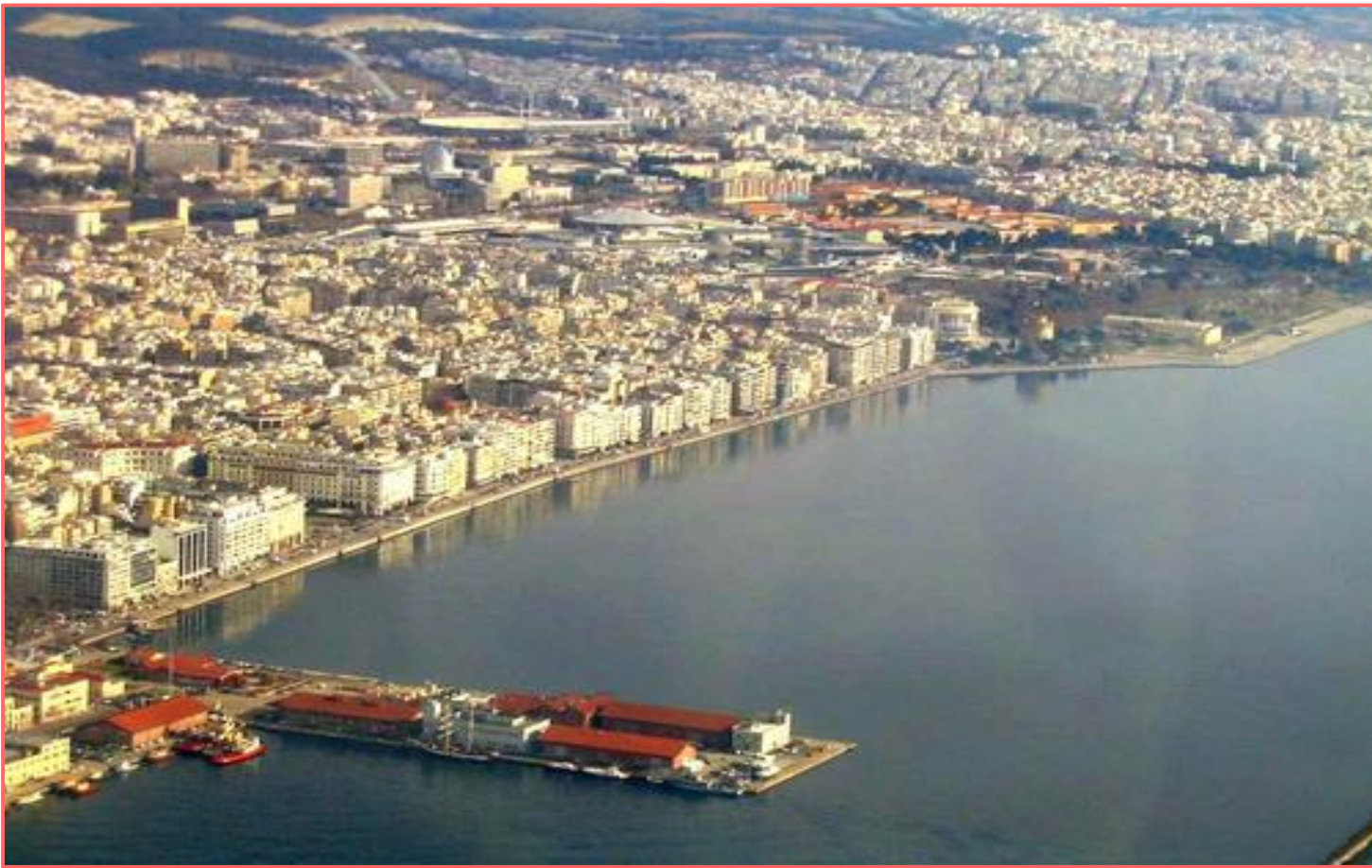
Pier A of the Port of Thessaloniki
